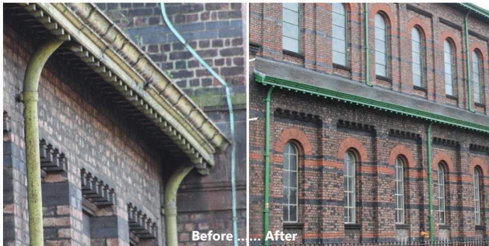
Thankfully we were able to find some undamaged patches of the original paint in normally-inaccessible places and from these three test patches were prepared of the closest shades of green available today. Once these dried we picked the "winner" which can be seen by anybody passing the church now that the scaffolding has come down.
